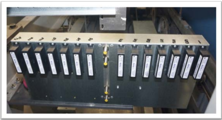
Figure 2.10: Typical Selector Box Installation
