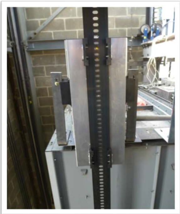
Figure 2.3: Typical Selector Installation
